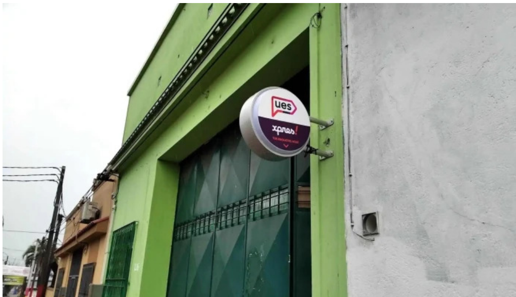
Pick up center ues rivera exterior
