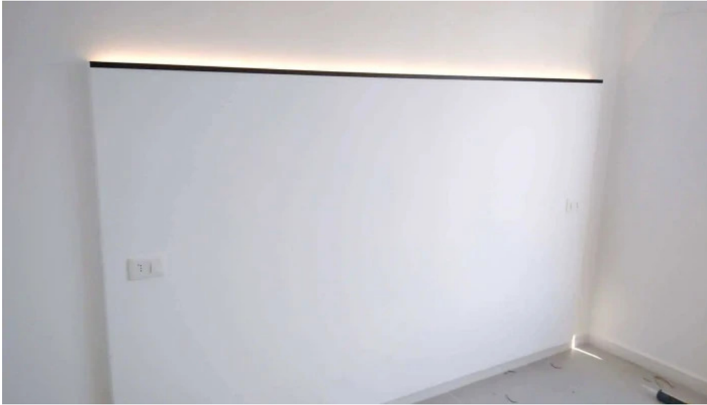
Electricista palermo interior
