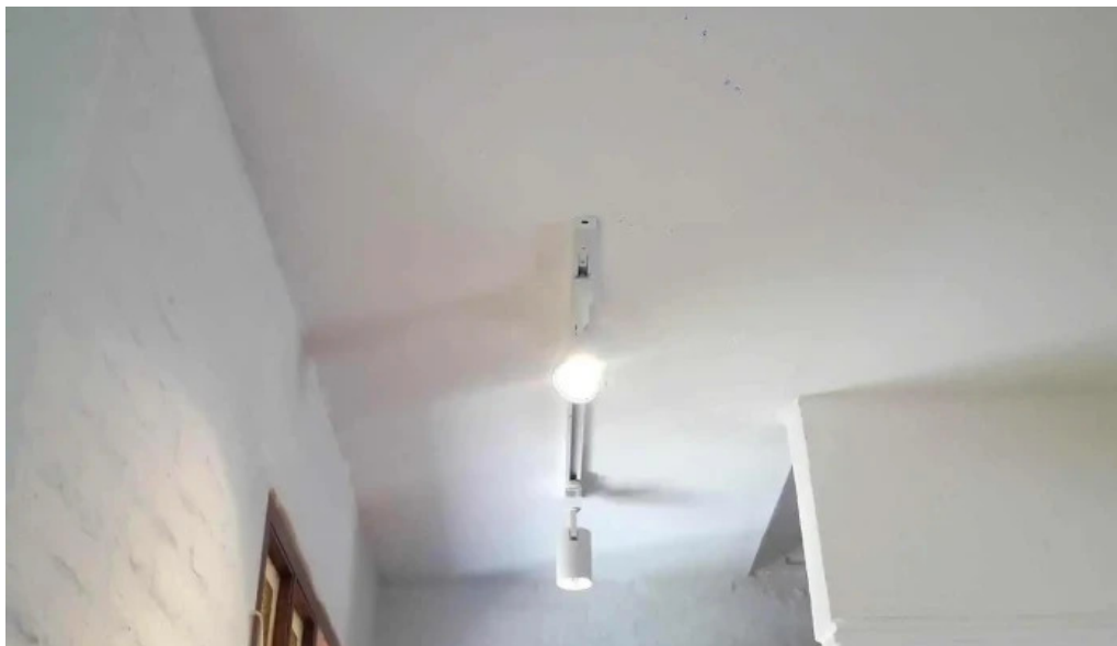
Electricista andres interior
